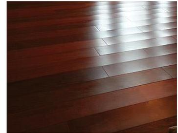
Bamboo floors that lose too much moisture can gap. Gapping occurs between floor boards. Gaps can vary in size and are considered normal if they appear and disappear during seasonal changes in humidity. Gaps are not considered normal if they are large or do not close during more-humid months.
